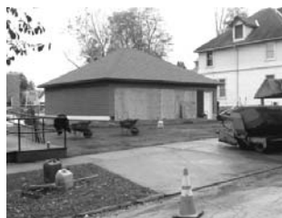
New Parking Lot ✓
